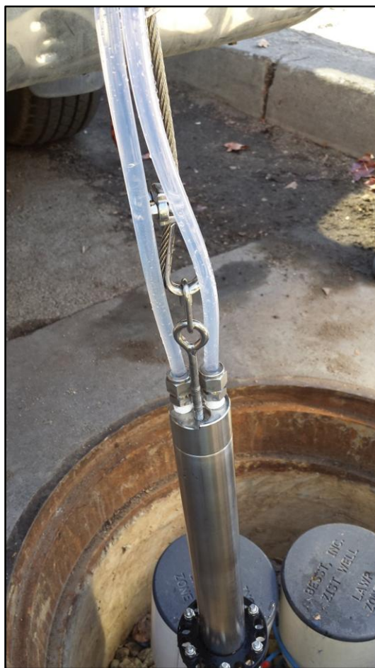
Figure 2- Stainless Steel Panacea P200 being deployed into a nested monitoring well in North Hollywood, CA. Tubing is 3/8" OD FEP bundled with 3/16" stainless steel support cable. The docking cage is located at the bottom of the photo.
